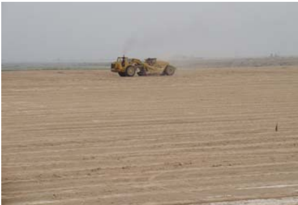
Figure 60. Southern Agricultural Region, land leveling for irrigation development in progress.
