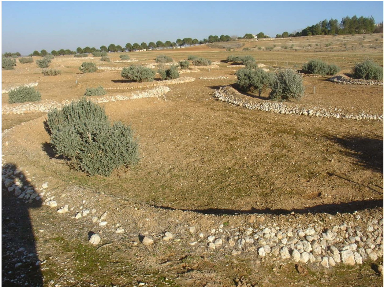
Figure 3. Semi-circular bunds, reinforced with stones, at the IWLMP Water Harvesting Site, ICARDA
