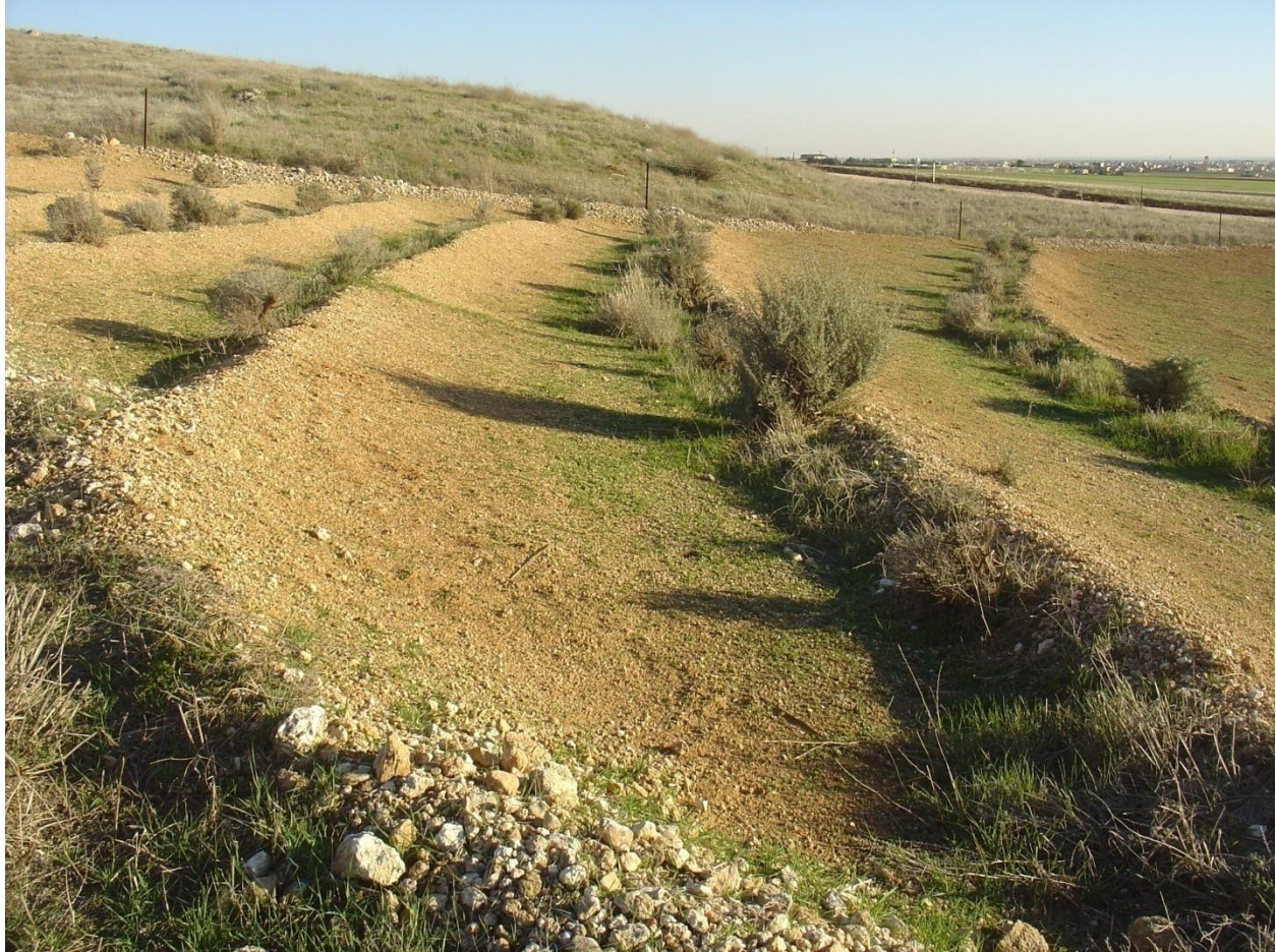
Figure 1. Contour ridges at the IWLM Water Harvesting Site, ICARDA, Tel Hadya
