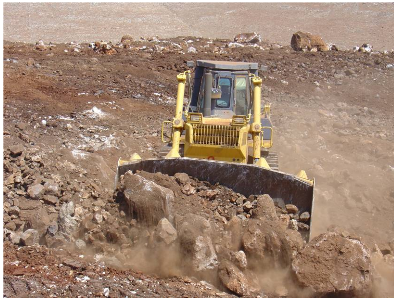
Figure 22. Initial clearing of the surface rocks
