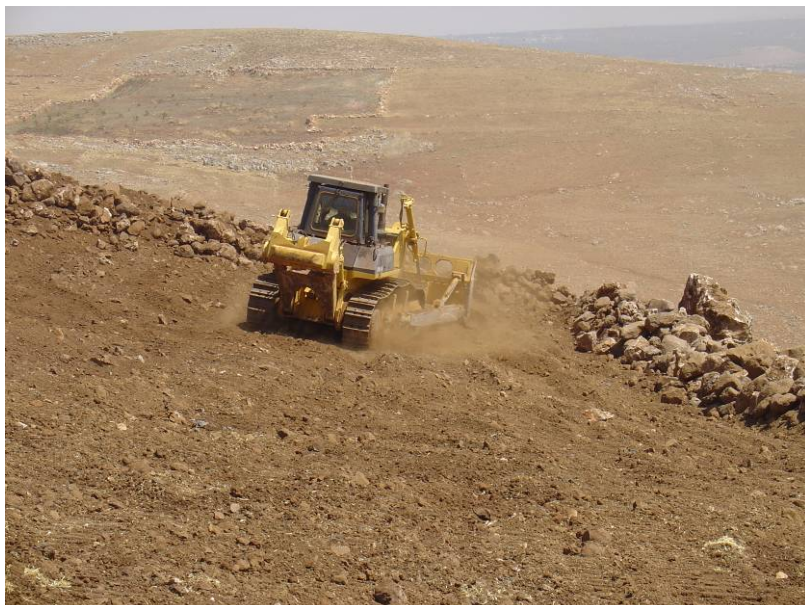
Figure 24. Piling up the rocks at the field edges
