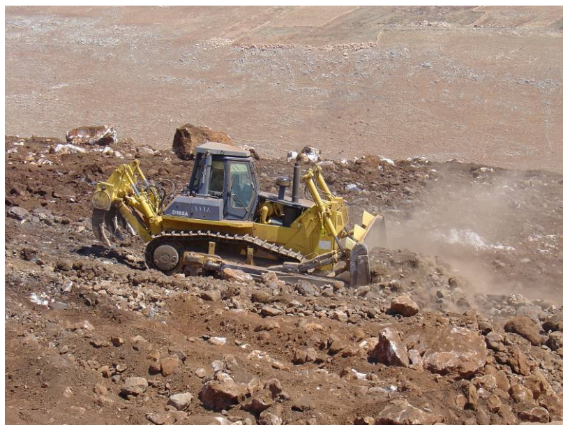
Figure 23. Ripping the subsoil to bring rocks to the surface
